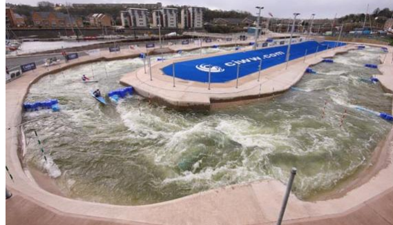
Completed canoe slalom and white water rafting facility
