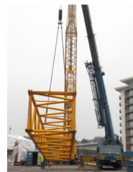
Section of the UK’s largest mobile crane
