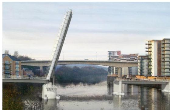
Pont-y-Werin Bridge open
