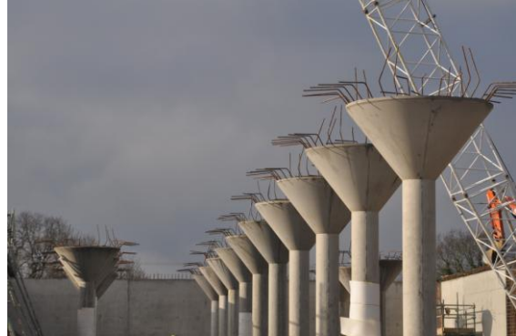
Internal reinforced concrete columns
